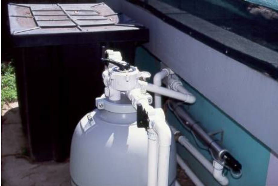
Three types of filtration- Mechanical (Grey pond filter), Biological (black tub with dense matting) and UV Clarification/Sterilisation (Stainless steel tube)
